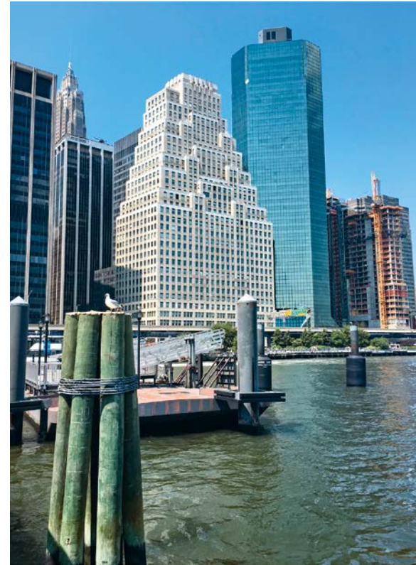
120 Wall Street (© Ekkehard Muther)
